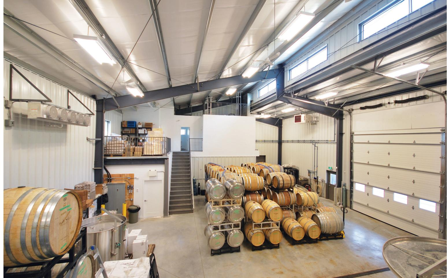
to get involved with another Norsteel project," says Shane Kennedy, branch manager of the Kelowna ASSA ABLOY office. "We were tasked with the fabrication and installation of a 15' x 16' commercial-grade, steel-insulated overhead door. For optimal thermal efficiency, we provided a door with polyurethane-injected sections and for natural light and transparency, the door featured four double-pane clear-tempered windows at eye level."
